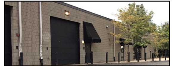
The Production Center, located at 601 15 th Street, New Brighton
